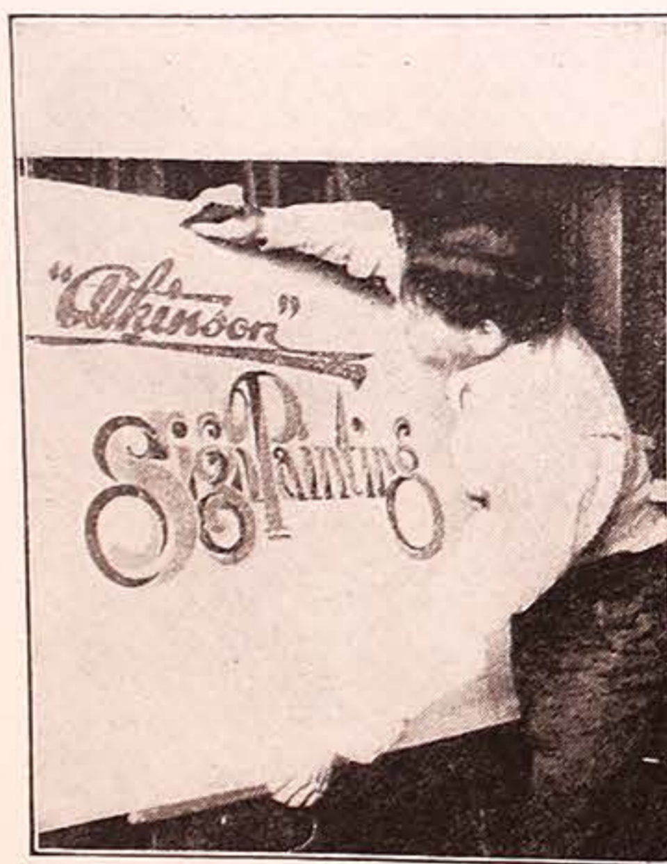
FIG. 17. SHOWING LINES DRAWN WITH TAUT STRING.
